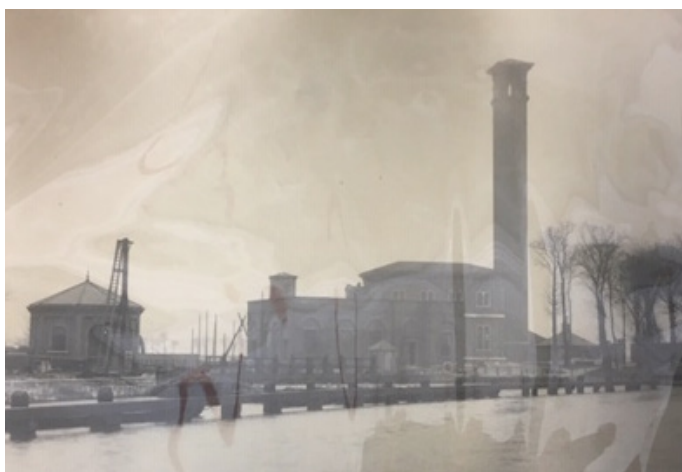
Fig 2.2 The East London Waterworks
