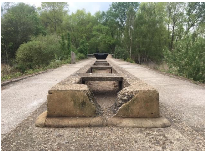
Fig 5.1 Contemporary Photo of the Filter Beds Character Area.
